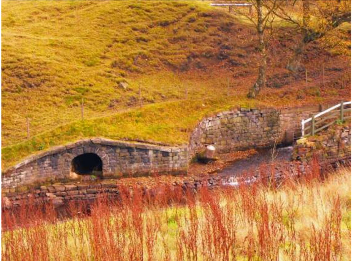
**Fig 3 - Rochdale Canal, Summit Level – left hand opening supply 'from moor top' reservoirs - right hand flow from “level drain” (Hollingworth Lake)**
