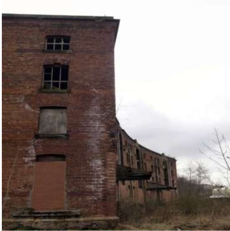
Fig.2: Clegg Street Warehouse - end elevation.
